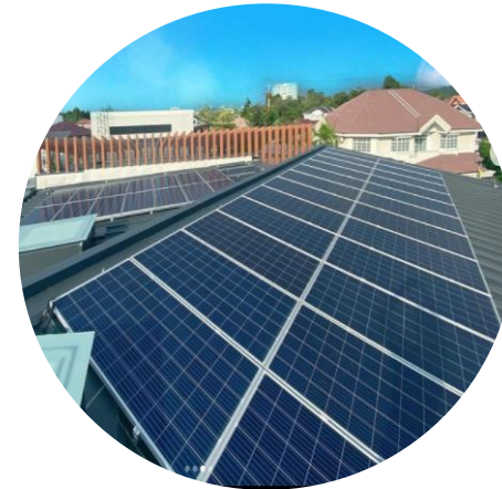
SYSTEM 30KWP 90 buah panel
